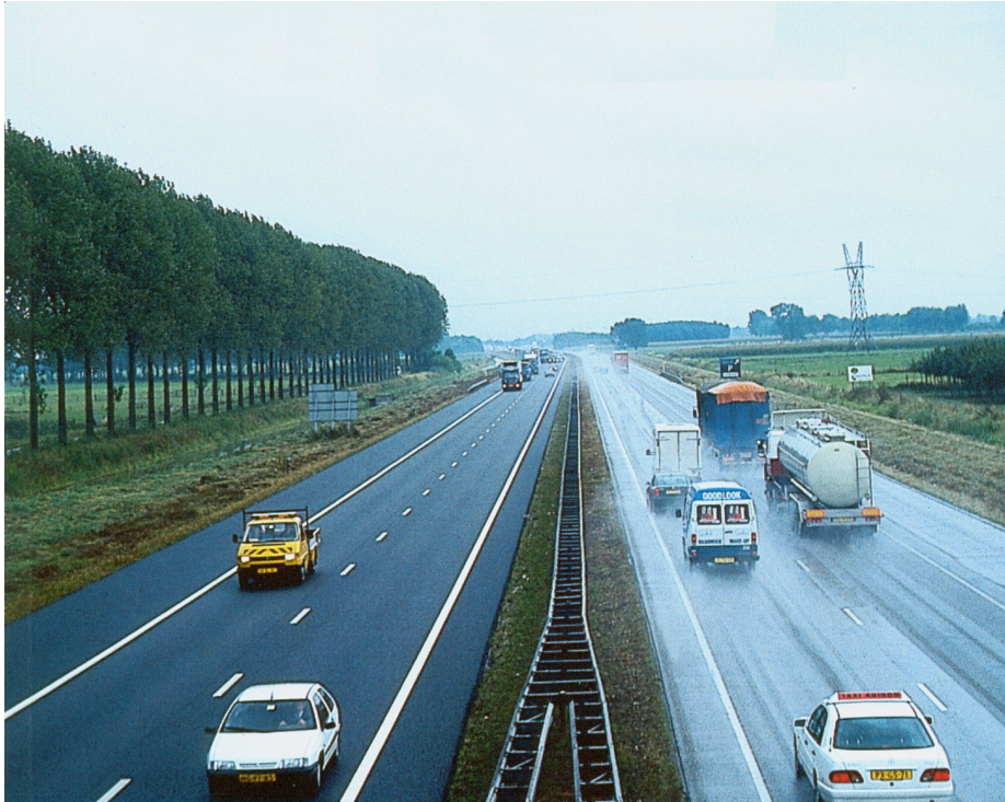
Figure 2.12. – Effect of rain on Open Asphalt Concrete (left) and Closed Asphalt Concrete (right)
