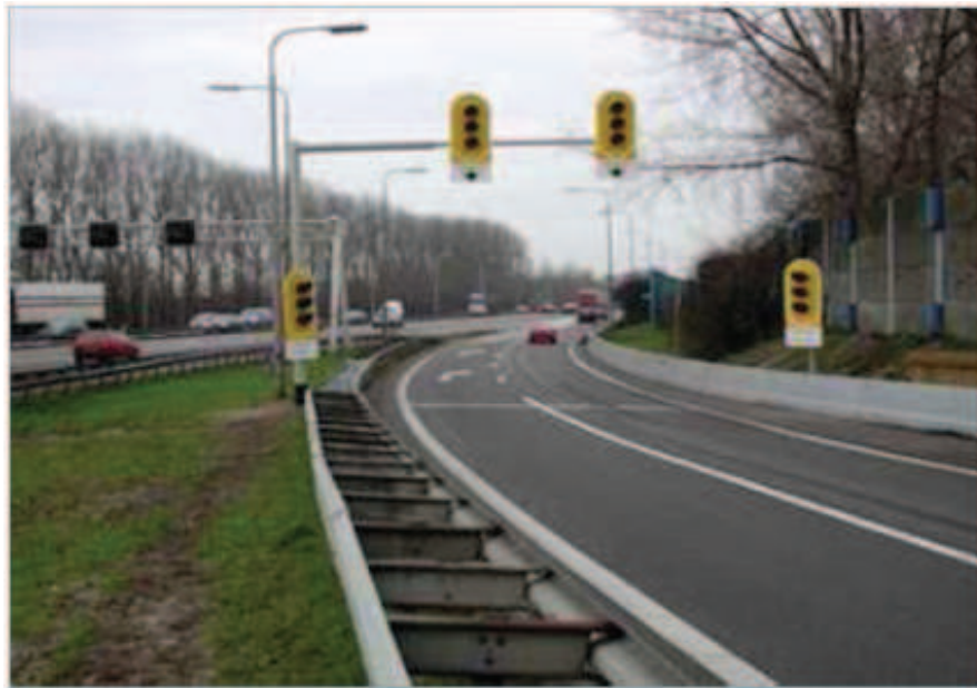
Figure 2.2: Ramp metering system in the Netherlands, A2 Maarssen-oost (Middelham and Taale, 2006)
