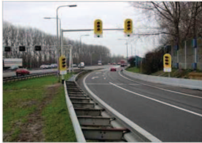
Figure 1.1: Ramp metering system in the Netherlands, A2 Maarssen-oost (Middelham and Taale, 2006)
