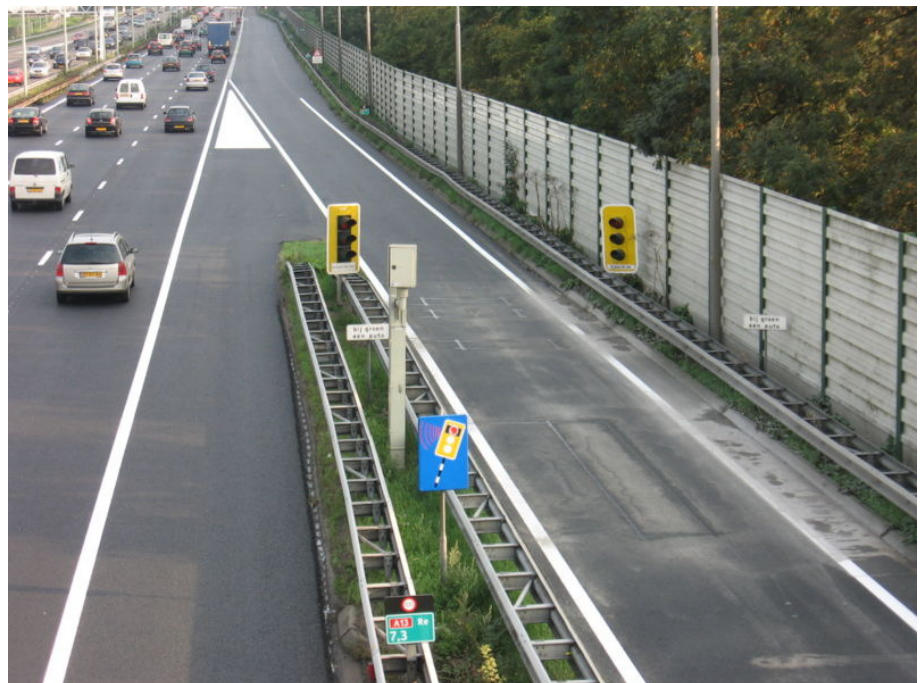
Figure 1.2: Ramp meter at the A13 Delft North on-ramp
